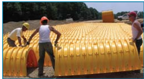
Lightweight Chambers Can Be Easily Installed By Two People
