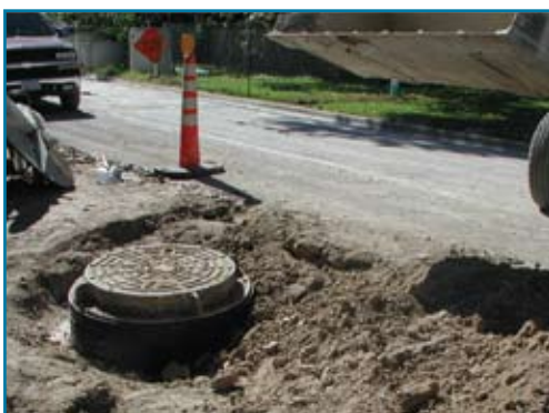
Manhole Frame & Cover Installed After HDPE Adjusting Rings Are Added
