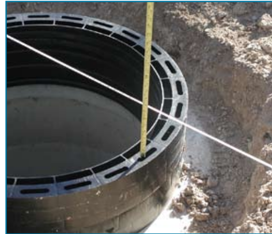
HDPE Adjusting Rings Are Added To Bring The Manhole To The Proper Grade
