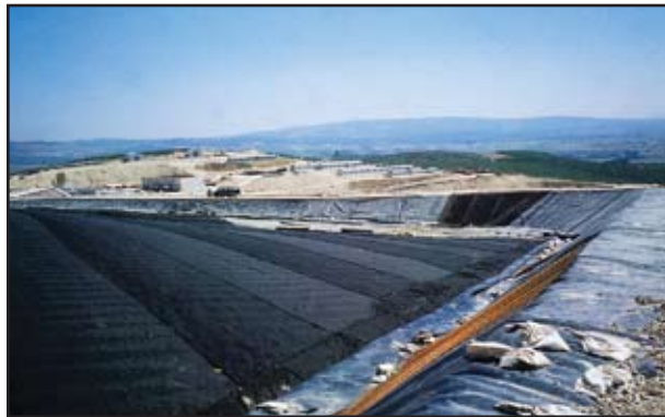
Nonwoven Geotextile is Used as a Cushion Under the Geomembrane Liner of This Landfill
