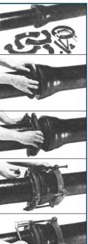
Clean pipe joint and bell face thoroughly. Caulked joints should not have caulking extending beyond the bell face. If recessed more than 1/8", face with lead wool or other suitable material if possible.
