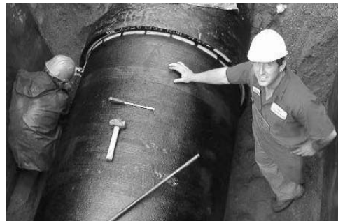
Richard Gowen of Gowen Excavating
