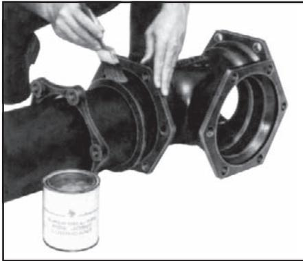
**1. Clean bell and plain end and lubricate gasket with pipe lubricant. The joint area must be free of dirt.**
