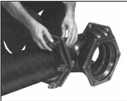
**3. When gland is in position, insert bolts and partially tighten with fingers.**
