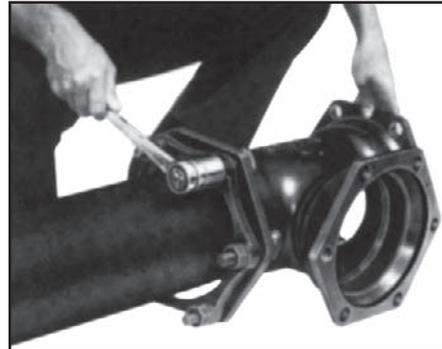
**4. Tighten bolts to the normal range of bolt torque [75-90 ft pounds] while maintaining approximately the same distance between the gland and the face of the socket.**
