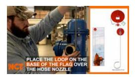
3. Replace the hose nozzle cover and tighten it down against the flag base loop.
