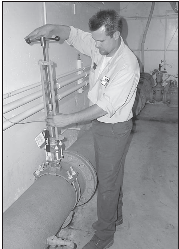
MBS technician installing a flow meter
