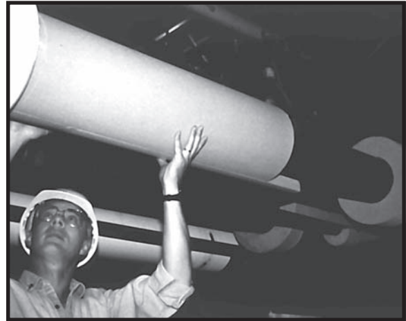
Shown Being Installed on Interior Piping; Also Recommended for Underground Applications
