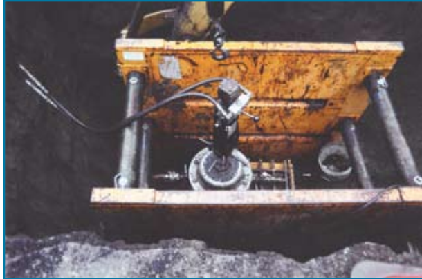
EJP Service Department Installing a QuikValve™
