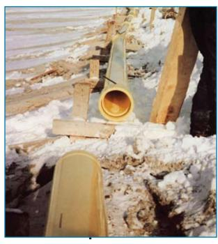
CertainTeed Yelomine PVC Pipe is made from a special formulation of Polyvinyl Chloride, Type 1, Grade 1, 2000 psi design stress material, Class 12454B in accordance with ASTM D-1784. The Yelomine PVC formulation contains additional impact modifiers and ultraviolet inhibitors to give it higher impact strength over a longer period of time.
