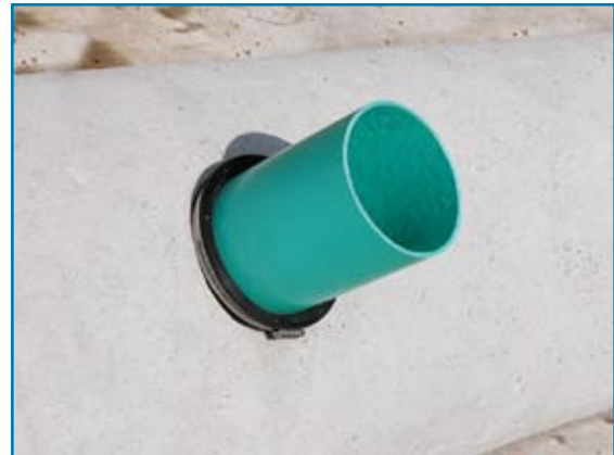
SDR 35 Pipe Connected to Concrete
