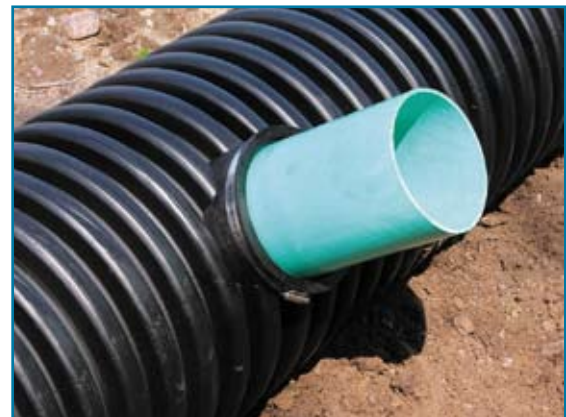
SDR 35 Pipe Connected to Corrugated Polyethylene Drain Pipe
