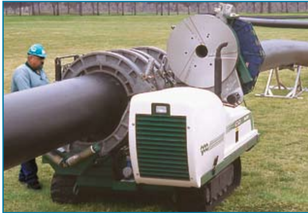
Fusion joining of HDPE pipe
