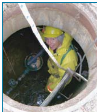
Confined space meter change-out installation. Technician is wearing a harness with gas detector and safety equipment.
