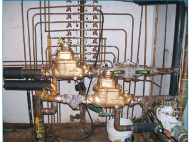
New Sensus Compound Meters are installed.
