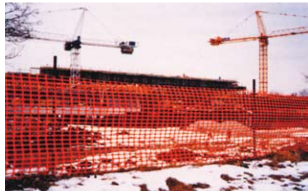
Construction Fence Helps Keep Job Sites Safe
