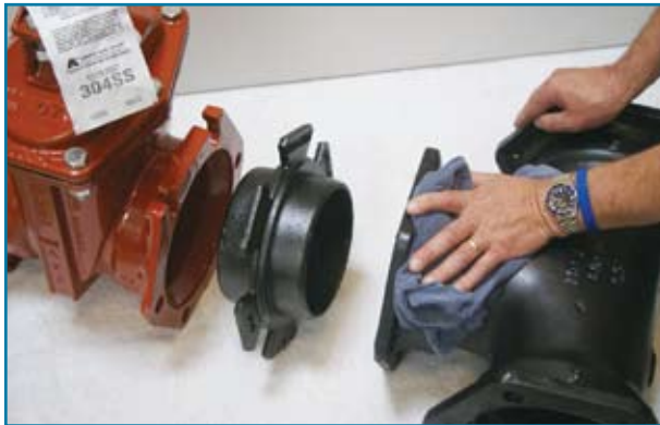
Clean Parts and Install Gaskets
